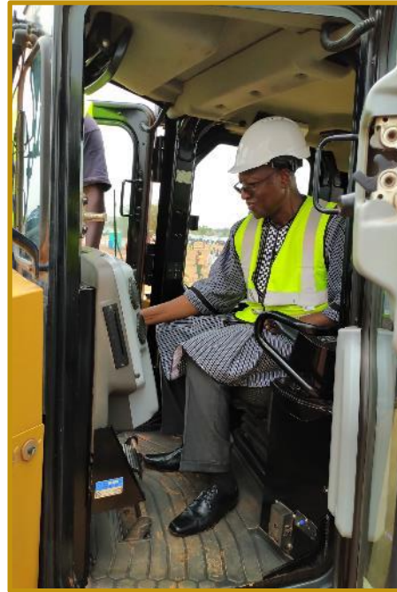
Burkina Faso Prime Minister, H. E. Christophe Dabiré starts the ceremonial bulldozer as a symbolic first shovel of the RAP construction
